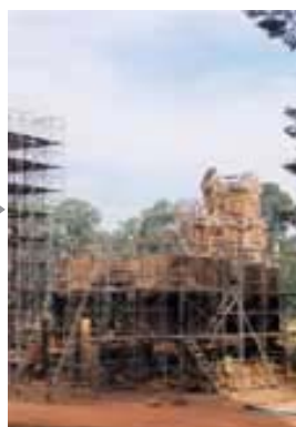
Dismantling Process of the N1 Tower of Prasat Suor Prat
