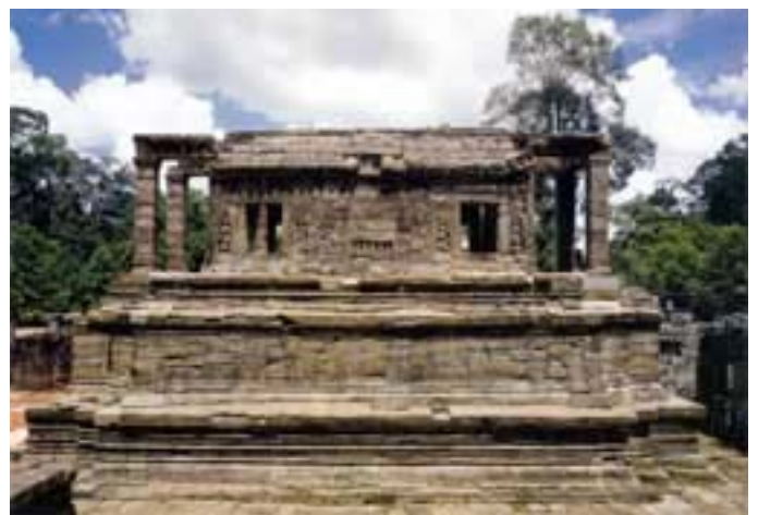
修復後 After Restoration
