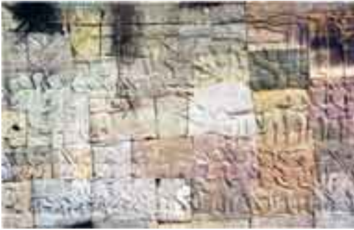
Pl. 2.6-1 The gray to yellowish brown sandstones used for the Outer gallery of Bayon. The size and shape of the sandstone blocks are variable and the stacking of the blocks seems to have been performed without a plan.
