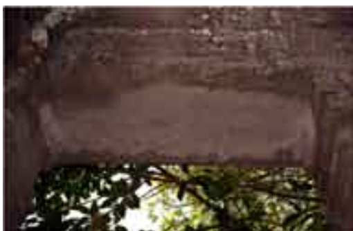
Pl. 2.6-4 The exfoliation due to crystallization of calcite in the under bed of the architrave in the Outer Gallery (East Entrance) of Bayon.
