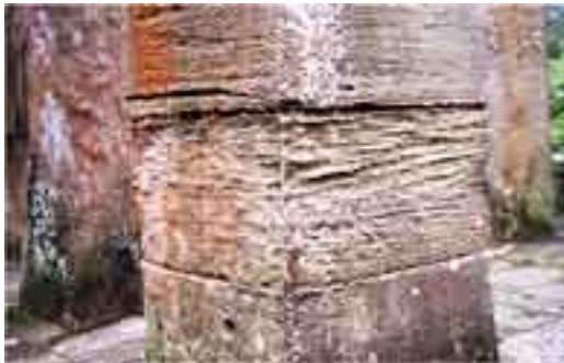
Pl. 2.6-10 Emphasized bedding planes due to tafoni in the pillar in the southeast corner building of the Outer Gallery of Bayon.
