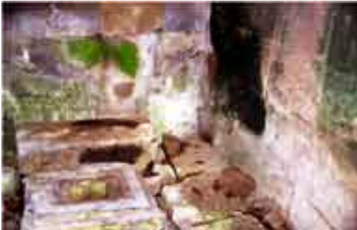
Pl. 2.6-3 The exfoliation of the sandstone blocks by salt weathering due to bat excrement in the lower part of the inner wall of the Tower 7 in the central part of Bayon.
