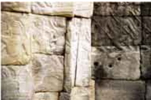
Pl. 2.6-7 Crack along the bedding plane in the gray to yellowish brown sandstone block with the vertical bedding planes in the Outer Gallery (north side) of Bayon.
