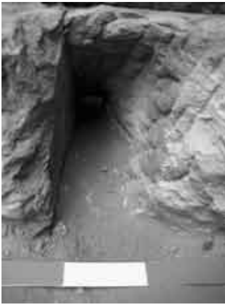
Pl. 2.8-7 Drain G-7, Chisel traces (additional drain).
