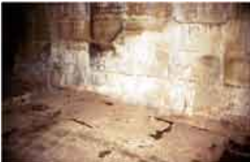
Pl. 2.6-2 The exfoliation of the sandstone blocks by salt weathering due to bat excrement in the lower part of the inner wall in the Inner Gallery (west side) of Bayon.
