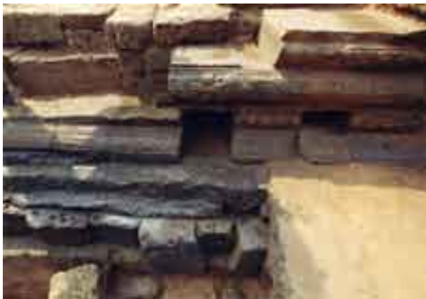
Pl. 2.4-7 "Culvert" exit found on the wall of the Outer Gallery platform, viewed from the north. 外回廊基壇の壁体で検出された暗渠排水溝出口〔北から〕.
