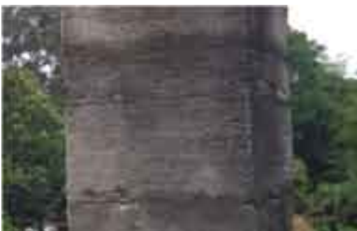
Pl. 2.6-8 Cracks along the bedding planes in the pillar constructed with sandstone blocks with the horizontal bedding planes in the Northern Library of Bayon.
