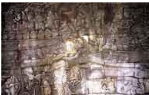
Pl. 2.6-12 Detachment of relief due to heterogeneity of the sandstone block in the Outer Gallery (in the east part of the south side) of Bayon.
