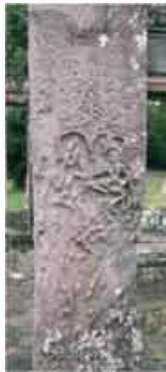
Pl. 2.6-9 Reliefs of dancing Apsaras on the pillars in the southeast corner building of the Outer Gallery of Bayon. (a) intact Apsaras and (b) weathered Apsaras due to tafoni.
