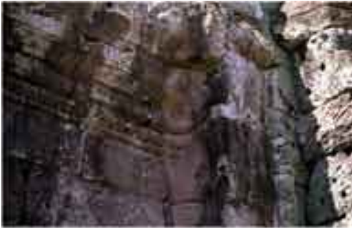
Pl. 2.6-5 Holes formed in the reentrant due to crystallization of calcite in the West Tower on the cruciform platform of Bayon.
