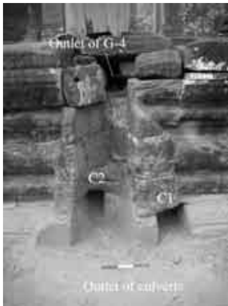
Pl. 2.8-14 Drain G-4 and two culverts below.
